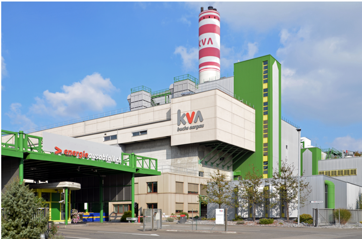
Photo 1: Working together cost-effectively for the environment. HZI will construct a hydrogen production facility at the Energy from Waste plant in Buchs, which is owned by the Aarau-Lenzburg Regional Waste Disposal Association. Messer Schweiz AG will add the facility's output to its product portfolio as green hydrogen.
